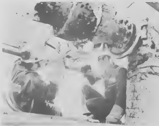
Holes are drilled in a flange before repairing a steam leak by injecting the sealing compound.
